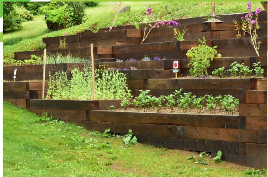
Treated wood is a good option to build garden beds as it is a cost effective and lasts longer than untreated wood.
